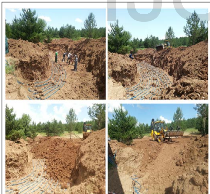
Fig. 3. Stages of placing the ground heat exchanger
